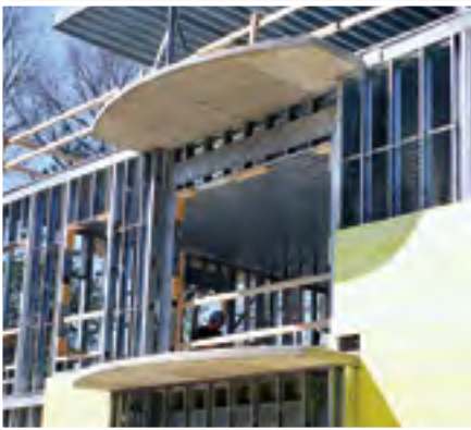
Cantilevered Formed-in-place Balcony
