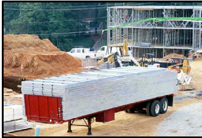
Figure 5.3- Prefabricated Wall Panel Delivery – Courtesy Infinity Structures
