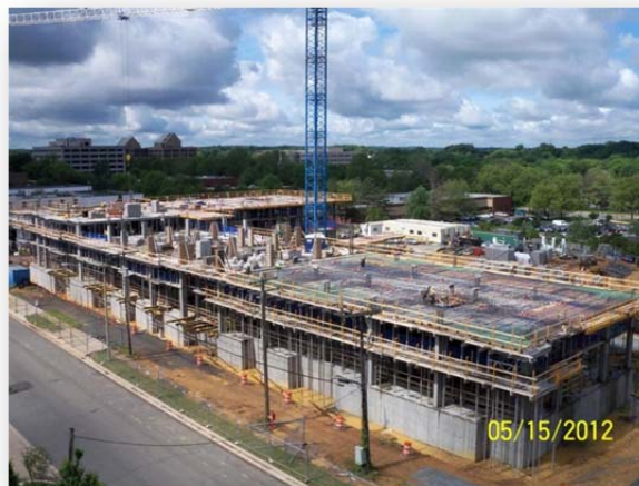
Figure 4.9: Cast –in-place – Courtesy of HITT
