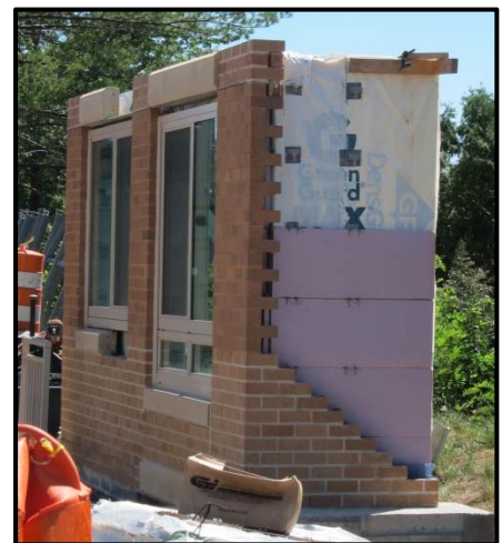
Figure 7.2 – Square 1400 Mock-up –Taken by Anthony Grab
